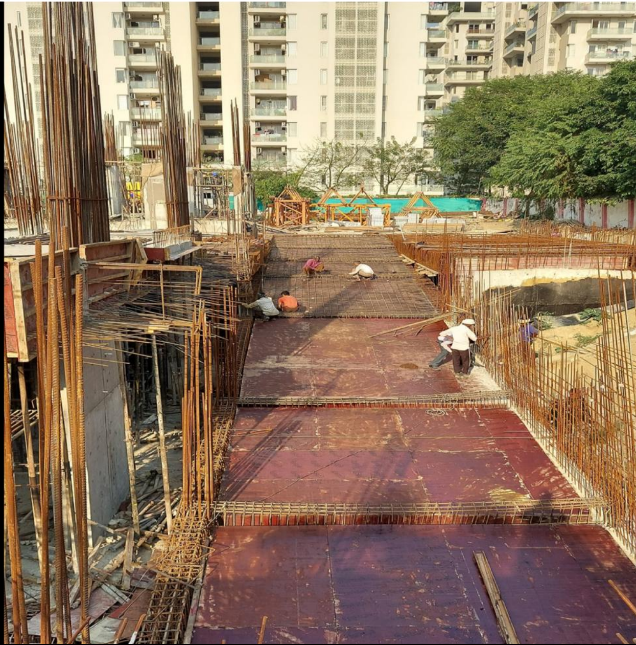
RAMP -2 , B1 TO GROUND FLOOR REINFORCEMENT IN PROGRESS
